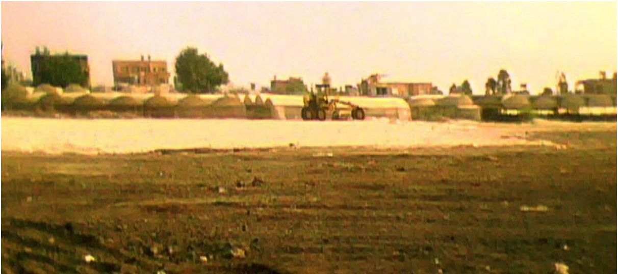
PICTURE 12: Clean up and shaping of the Kazanli beach
